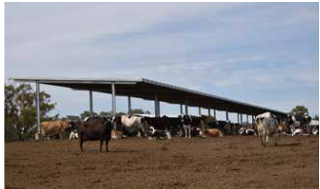
Figure 24. Centralised shade shelters at a dairy dry lot with a north-south orientation
