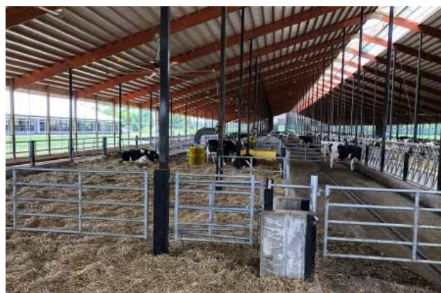
Figure 30. Deep litter pack – low bed retaining curb, water troughs, access from feed alley only
