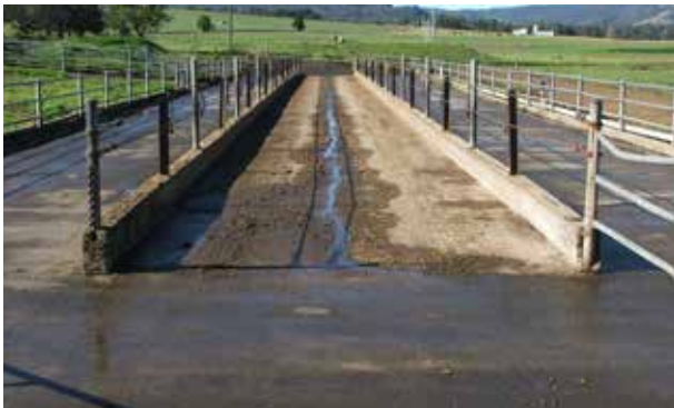
PMR fed out on fully concreted feedpad with nib wall, central feed alley
