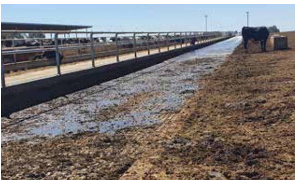
Flood washing of concrete cow feeding alleyways
