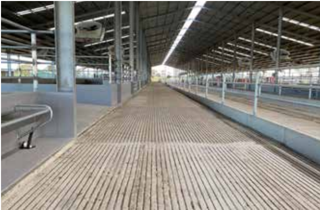
Figure 67. Concrete grooves on flooring
