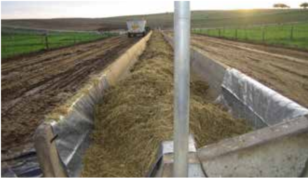
Formed earthen feedpad with concrete troughs
