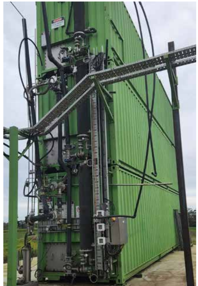
Figure 104. A Gekko Systems biodigester on a dairy farm at Bungaree
