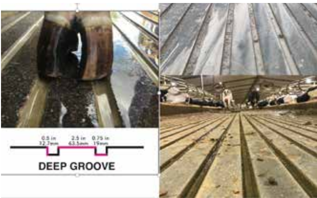
Figure 68. A deep groove pattern provides the best traction for cows
