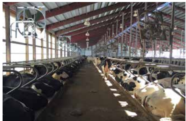
Figure 54. Two-row tail to tail freestall pen
