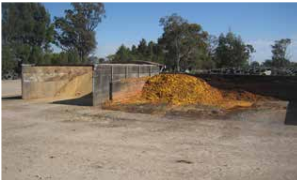
Concrete bunkers for storing by-products
