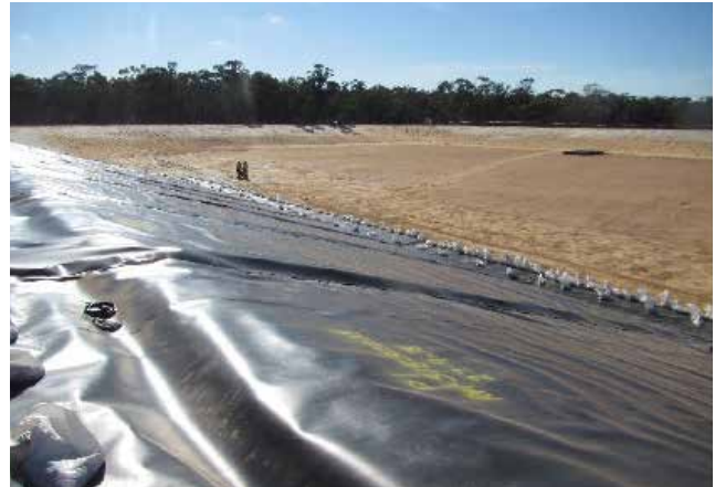
Figure 5. HDPE lining installed for impervious ponds in northern Victoria
