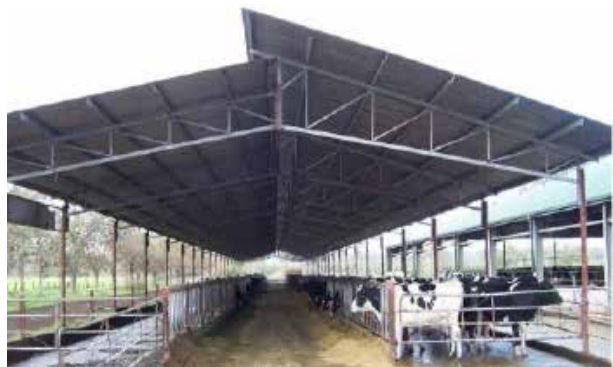
Concreted overlapping roofed feedpad
