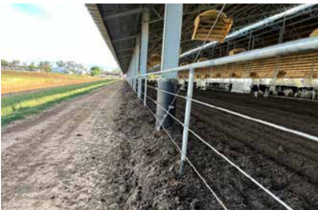
Figure 40. Eave overhangs can help minimise the amount of wind, precipitation, and sunlight entering the barn
