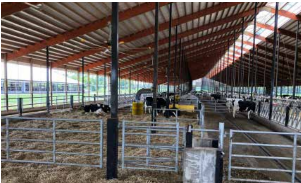
Deep litter pack – low bed retaining curb, water troughs, access from feed alley only
