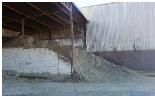
Figure 87. Design individual bays to cater for typical delivery truck volumes – store feed undercover
