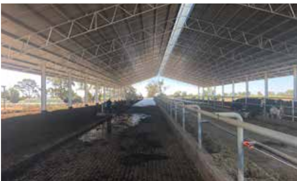
Concrete roofed feedpad with extended eaves for cattle loafing
