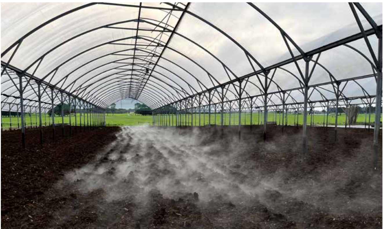
Figure 23. Redpath clear roofed deep litter shelter. Redpath shelters are steel framed with a flexible clear roof (polythene) membrane
