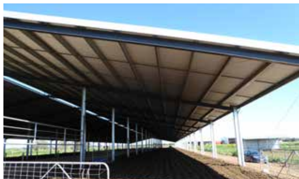
Concrete roofed feedpad with dry scrape feed alleys
