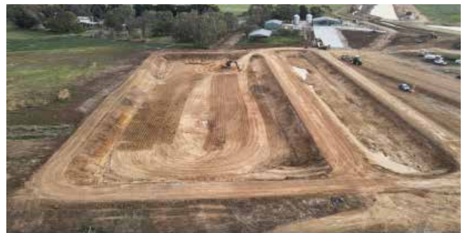
Figure 7. Construction of a an earthen feedpad and ponds
