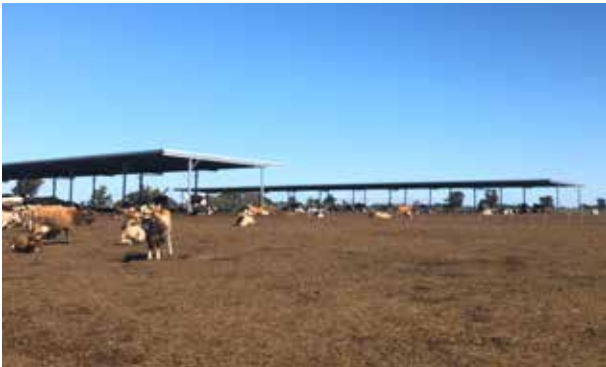
Shade shelters at a dairy dry lot with a north-south orientation
