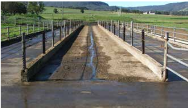
Concrete feedpad with separate drive and feed alleys
