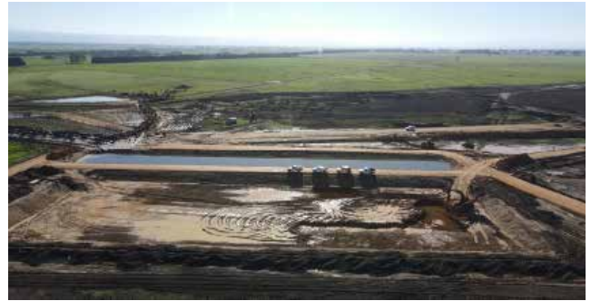
Figure 6. Construction of a an earthen feedpad and ponds – long view
